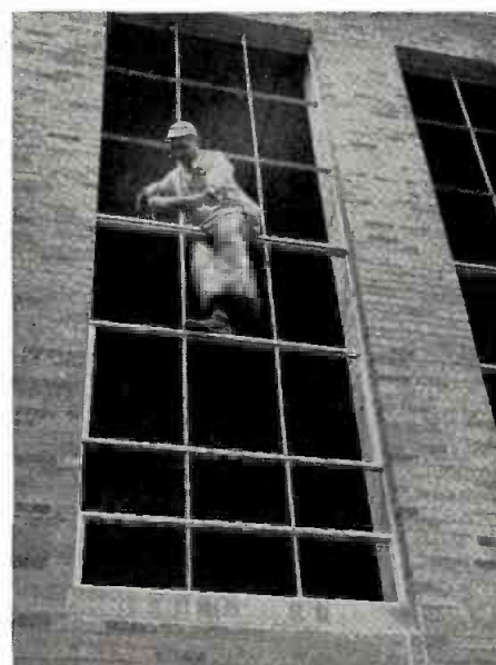
A Quarter Ton Of Glass must be supported by the sash in this convent-school. The sash is double glazed with stained glass on one side, clear glass on the other. Because of the great weight, and the high winds in the area, the authorities chose steel windows because they are so strong. For many years, United States Steel has furnished special rolled steel window sections for manufacturers all over the country.
